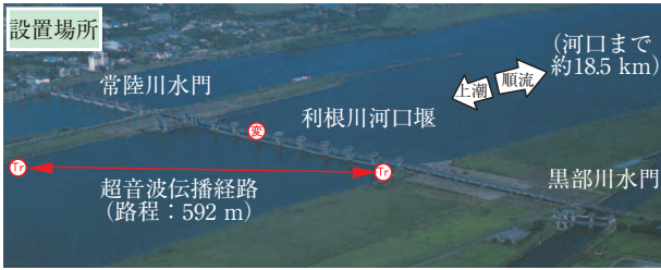
Fig. 4 Ultrasonic path layout at the Tone River Estuary Barrage
